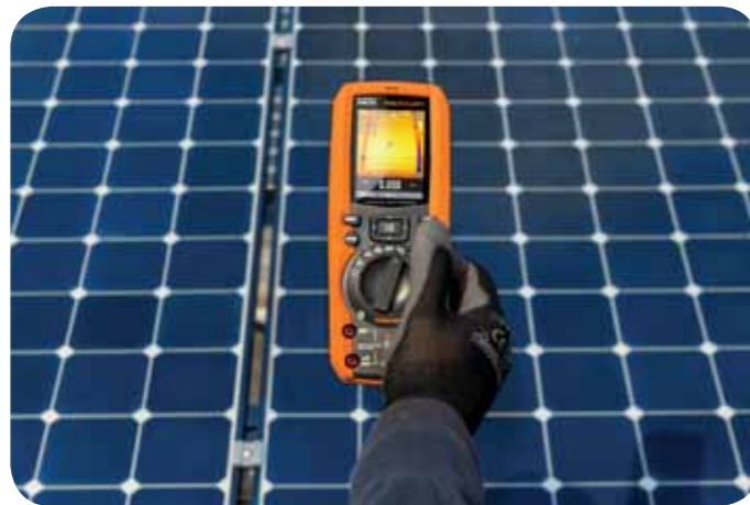
PV field thermography.
